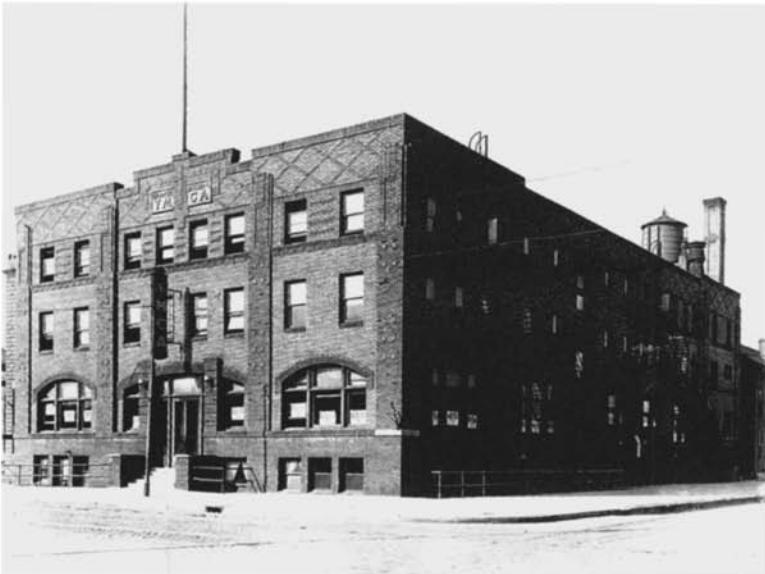
Fig. 1.8 Indianapolis's "Colored" YMCA Branch Building (built in 1912), where the National Youth Administration-sponsored LaVon Kemp Orchestra rehearsed. The signs in the windows state "Some Doings. Colored YMCA. ?" Photograph courtesy of Indiana Historical Society, Indianapolis.
