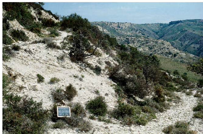
Fig. 3. Overgrown switchback ascent on the road between Coral Bay and Arodes, on the highway from Nea Paphos to Marion. This section was built at the end of the second century AD and engineered to Roman standards. Author’s photo, April 1991.
