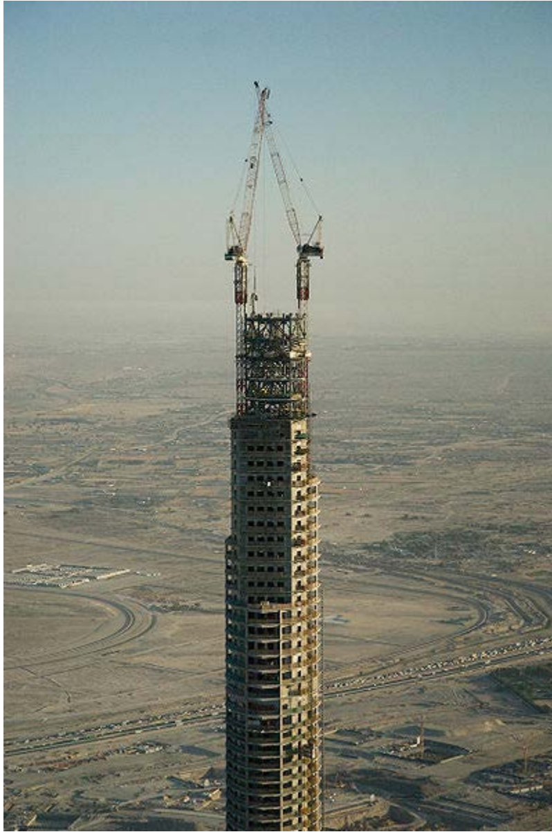
Aerial closeup of Burj Khalifa under construction in March 2008
