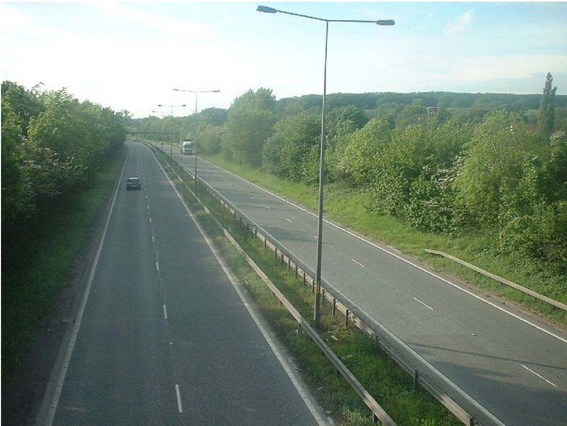
A typical British dual carriageway with central barrier on the A63(T) near Hull, England.
