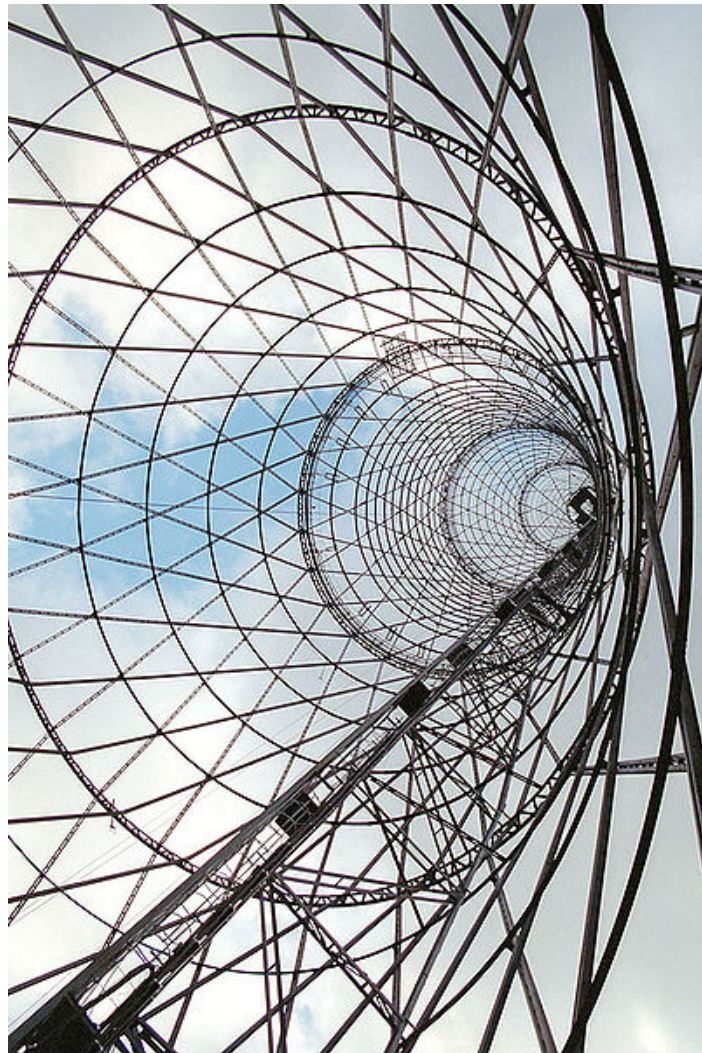
The gridshell of Shukhov Tower in Moscow. Currently under threat of demolition.
