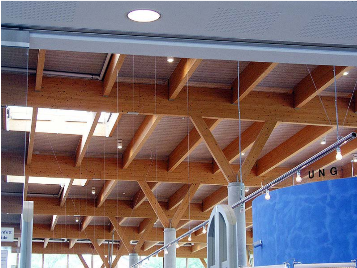
The roof of a library, Sweden.
