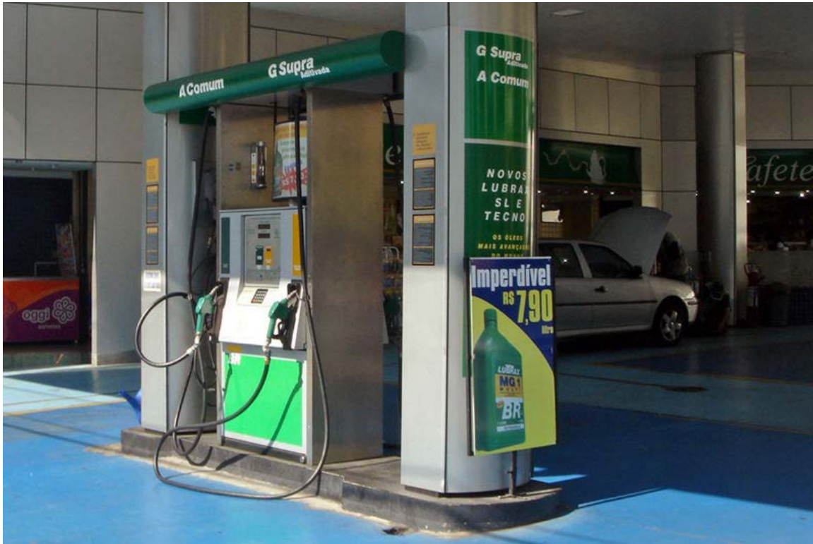
Neat ethanol on the left (A), gasoline on the right (G) at a filling station in Brazil
