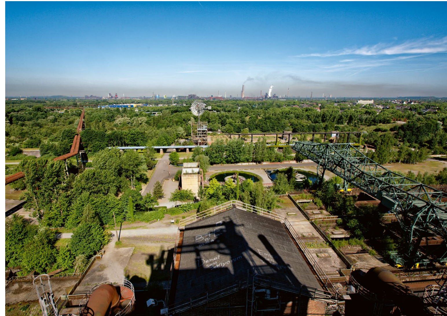
9 From a vertiginous height we look across giant coal and ore bunkers at the silhouette of the power plants and blast furnaces in the distance.
