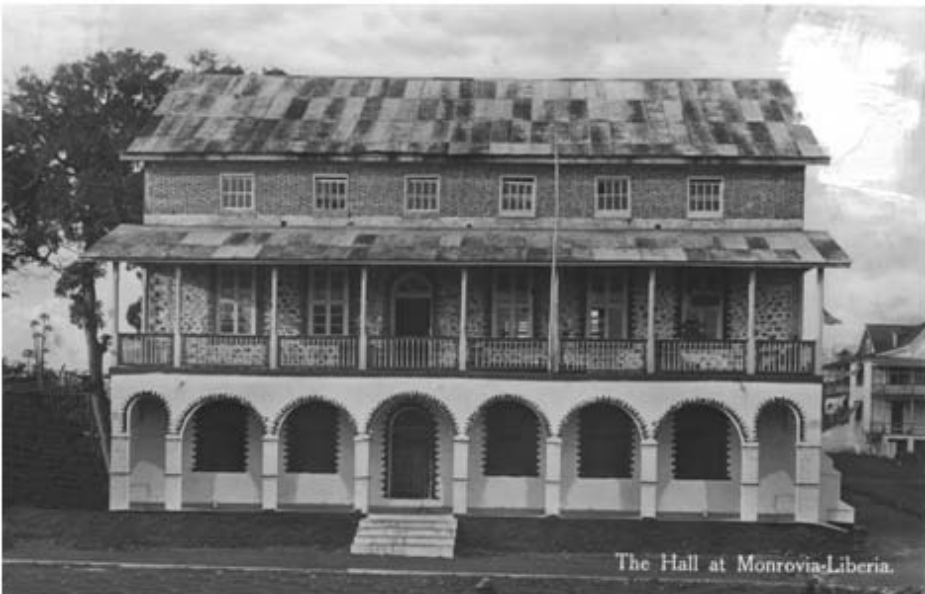
The Legislative Hall late 1920s by M. Dinklage, Jr. (The Hall at Monrovia-Liberia)
