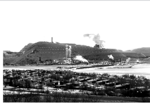
Fig. 1.8. Kirunavaara iron ore mountain, northern Sweden. The steeply dipping magnetite orebody was originally mined in an open pit on the left side of the hill. Today, extraction is underground. Reproduced by permission of LKAB.
