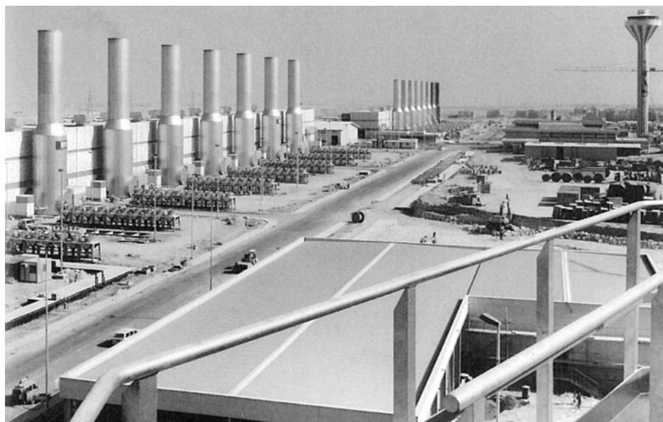
Figure 2-15 Riyadh 8, 800 MW – Gas turbine power station in Saudi Arabia © ABB
