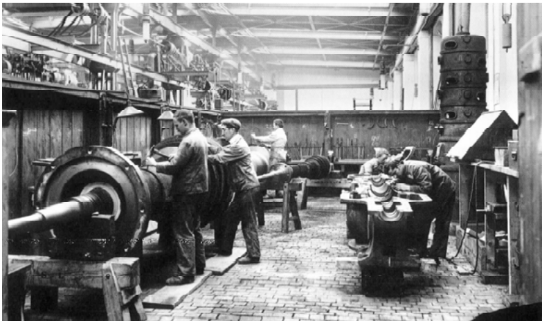
Figure 2-8 Steam turbine assembly, Baden ca. 1902 © ABB
