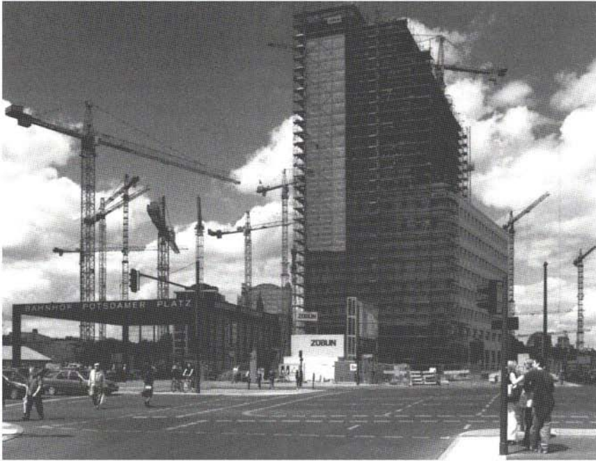
Figure 1: Cranes and construction on Potsdamer Platz , June 2002
