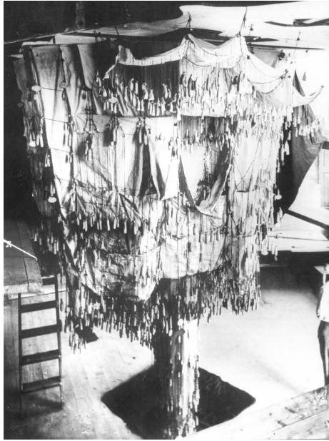
Fig. 1.2. Scale model for the Colonia Güell church
