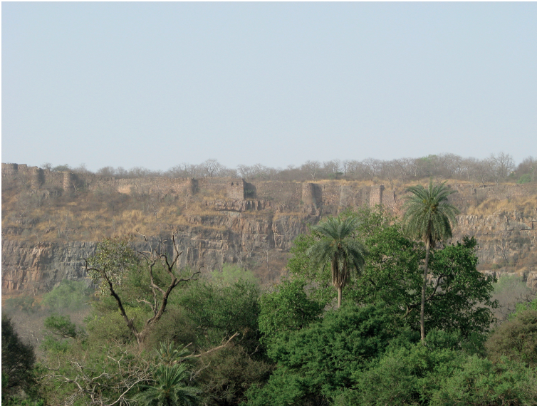
Fig 1: Outer wall of the fortress
