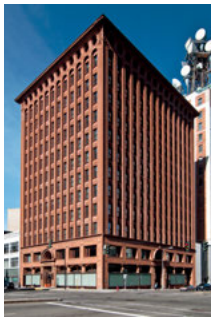
Adler & Sullivan's Guaranty Building in Buffalo, NY, USA, was completed in 1896. Some of the highly ornamental, complex elements have been recently recreated and replaced using hand-pressed molding techniques almost identical to the methods employed when the building was first built.
