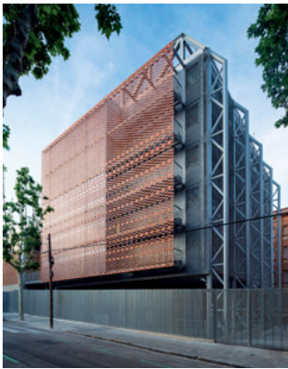
The extension of Antoni Gaudí's Teresianas School in Barcelona, Spain, designed by Picharchitects, features a facade composed of hollow ceramic extrusions. The so-called Flexbrick system features ceramic elements clipped onto a thin wire mesh to create a semi-transparent screen that filters light and views.
