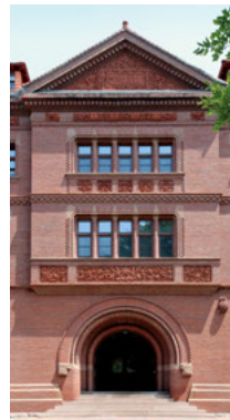
Sever Hall, completed in 1880, is an example of using terra cotta to "embellish" brick buildings in the Northeastern United States. Ceramics are used for highly ornamental elements only, and in combination with cut stone.
