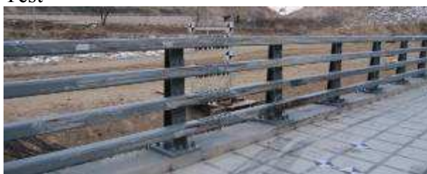
Fig. 12 Barrier Distortion and Shatter after Bus Impact
