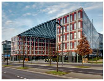
The roof geometry is generated by translating a transverse arc along a longitudinal rail (scaletrans surface). The gaps between the roof perimeter beams and the eaves of the building's two wings are closed with inclined panes of flat glass. This means of modeling makes it possible to surface the roof with transparent glass: rectangular panes of flat, laminated glass.
