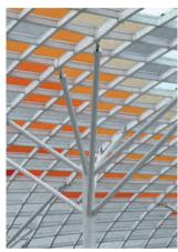
The treelike supports, spaced 15 to 25 m apart, reduce the spans within the canopy, which covers 35,000 m<sup>2</sup>—one of the world's largest free-form glazed roofs. Branching them allows the supports to be slenderer at the roof and shortens the spans in an efficient way.
