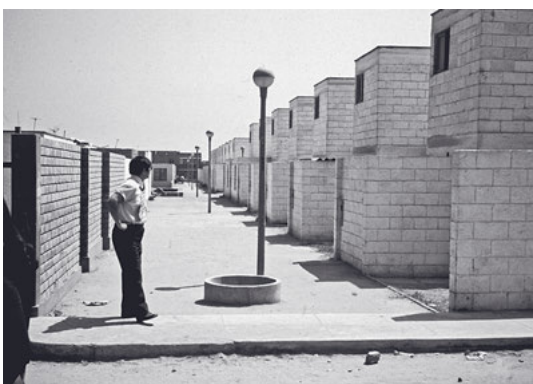
Maki at PREVI, low-cost housing project, Lima, Peru, 1972
