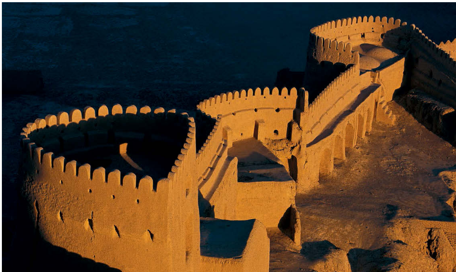
11. The view from the citadel of the eastern side of Bam's third curtain wall. Photo: 2001.
