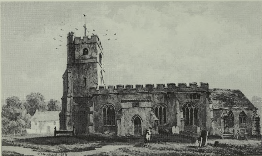
Plate 1. Harlington: South view showing the sundial on the porch (mentioned as early as 1686) and the windows in the chancel and belfry partially blocked up with masonry. The high level window in the south wall was blocked up in a C19th restoration of the church.
