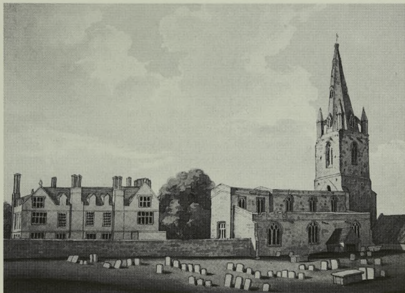
Plate 2. Harrold: View from the north showing Harrold Hall built in 1608–10 on the site of the old priory. Note the shortened chancel, and the north porch removed in about 1850.
