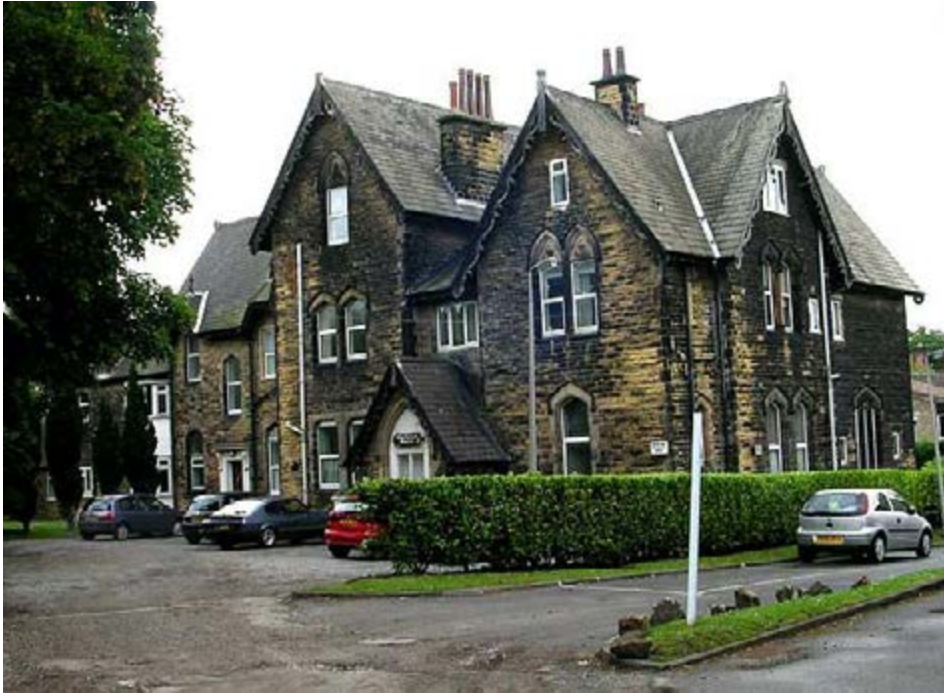
Figure 1.1: Weetwood House, Headingley.
