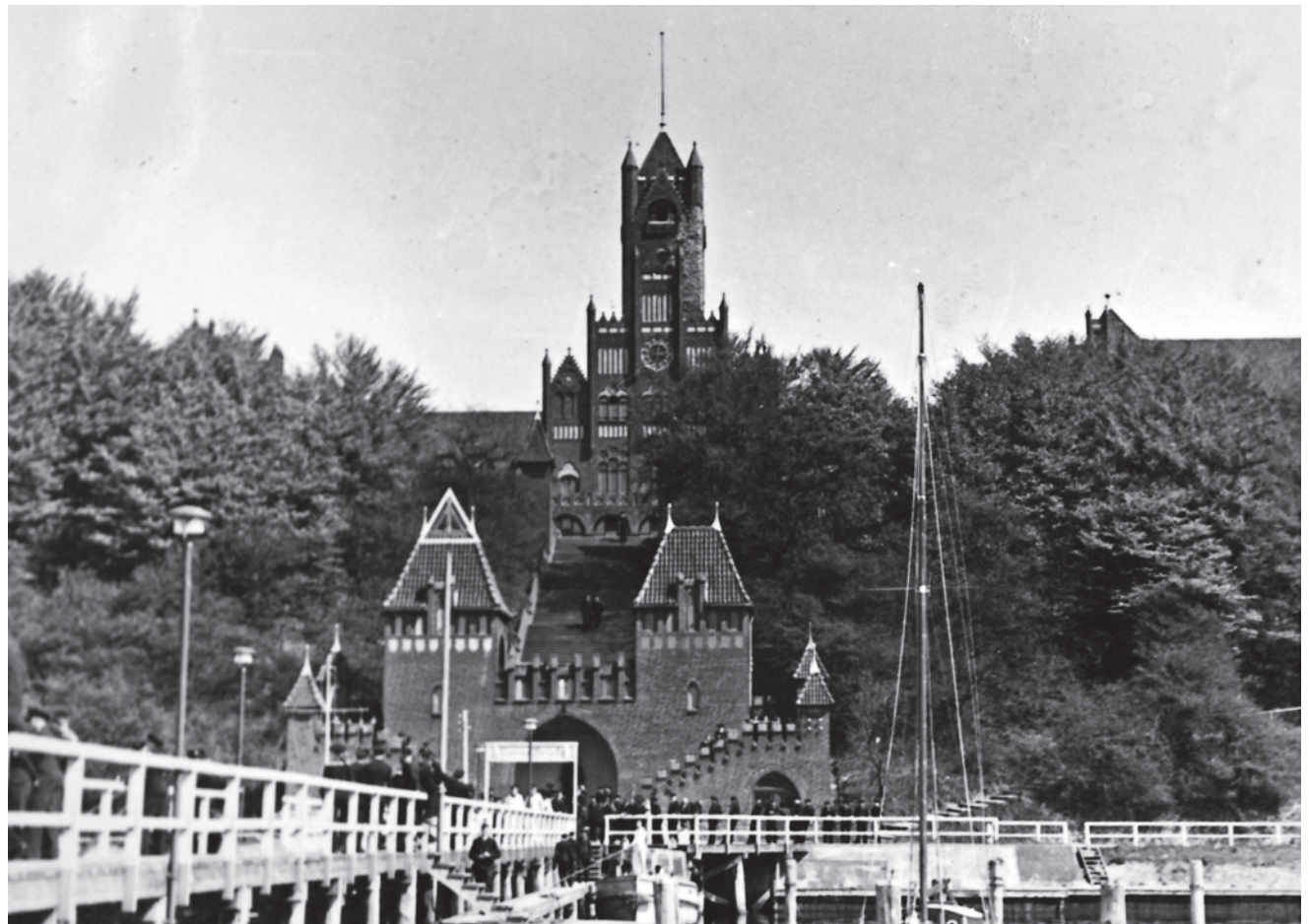
The Naval Officers' School – the Red Palace by the Sea – at Mürwik (Eckernförde) as seen from the water's edge. This impressive building was opened just a few years before the beginning of the First World War because the Naval Academy in Kiel, now occupied by administration for Schleswig-Holstein, could be expanded no further.
