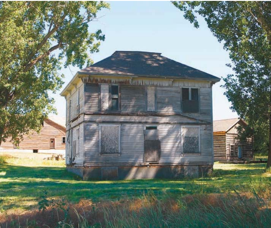
An unusual pyramidal rooftop caps this boarded-up two-story residence in Mayville, Oregon.
