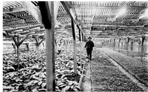
Early 20th-century wood-lath shade structures. Photos courtesy of Bob Beyfuss and Cornell Plant Pathology Herbarium.
