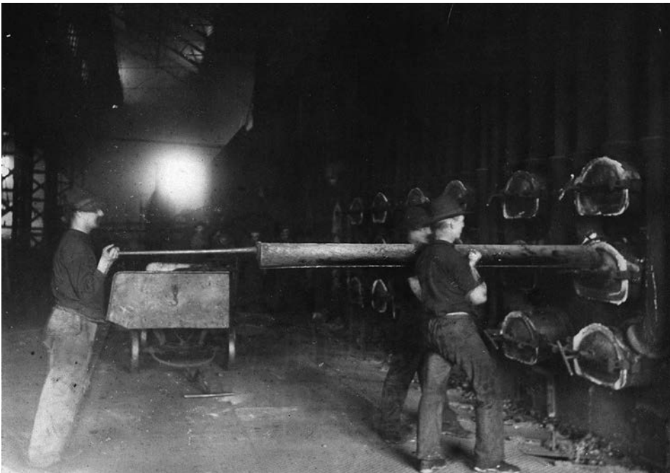
FIGURE 1.8 Interior of the Commercial Point retort house, showing stokers charging a retort in the 1880s.
