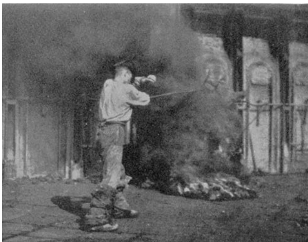
FIGURE 1.10 A 1936 photograph vividly depicting the drawing of a spent charge of red-hot coke into the retort house, amid a cloud of smoke and gas.
