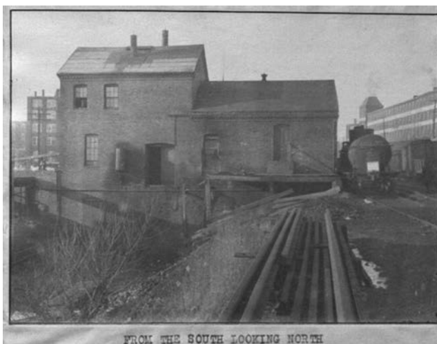
FIGURE 1.4 Exterior view of the Amesbury Gas Light Co. generator house. (Barber, Earl H. Report on the Amesbury and Salisbury Gas Company, January 5, 1920 . Baker Library Historical Collections, Harvard Business School. Earl H. Barber Papers, Vol 1 Case 14.)
