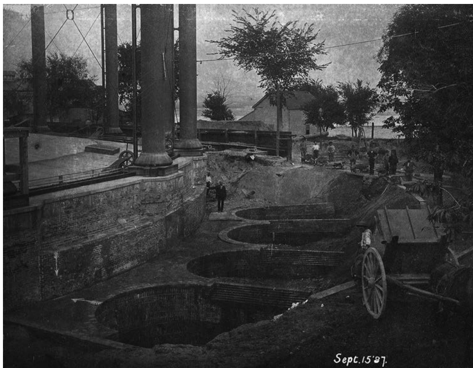
FIGURE 1.9 An 1887 image showing foundation buttresses for a gasholder at Commercial Point.
