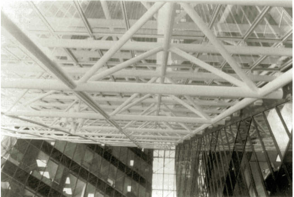
Fig. 1.1. Onshore applications of tubular structure. (a) Firth of Forth railway bridge, Scotland, 1880's. (b) Atrium space frame, Houston, 1980's.
