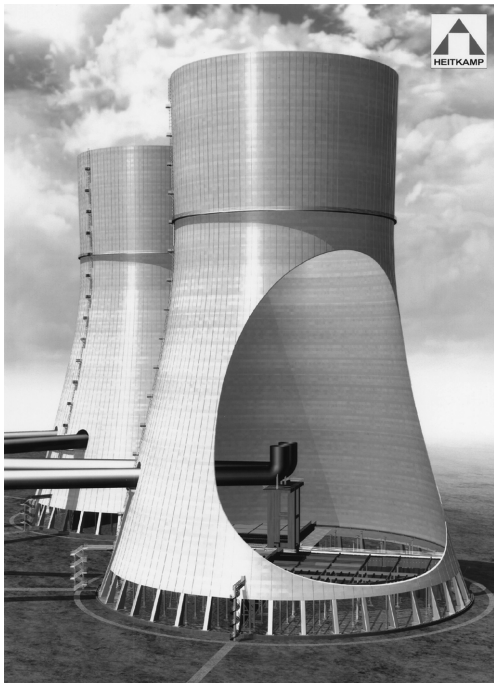
Figure 1. Natural-draught wet cooling-tower with cleaned gas intake system.
