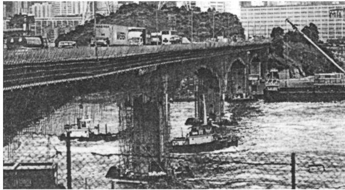
Fig. 6. The bridge under repair.
