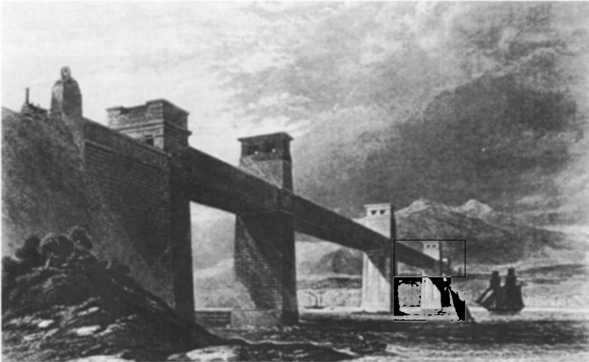
Fig. 1.1 Wrought iron box girders of 140 m span of Britannia Bridge, Wales, 1849; designed by Robert Stephenson. Lithograph from Cyclopaedia of Useful Arts by C. Tomlinson, 2nd edn, 1866. Photograph courtesy of Elton Engineering Books.
