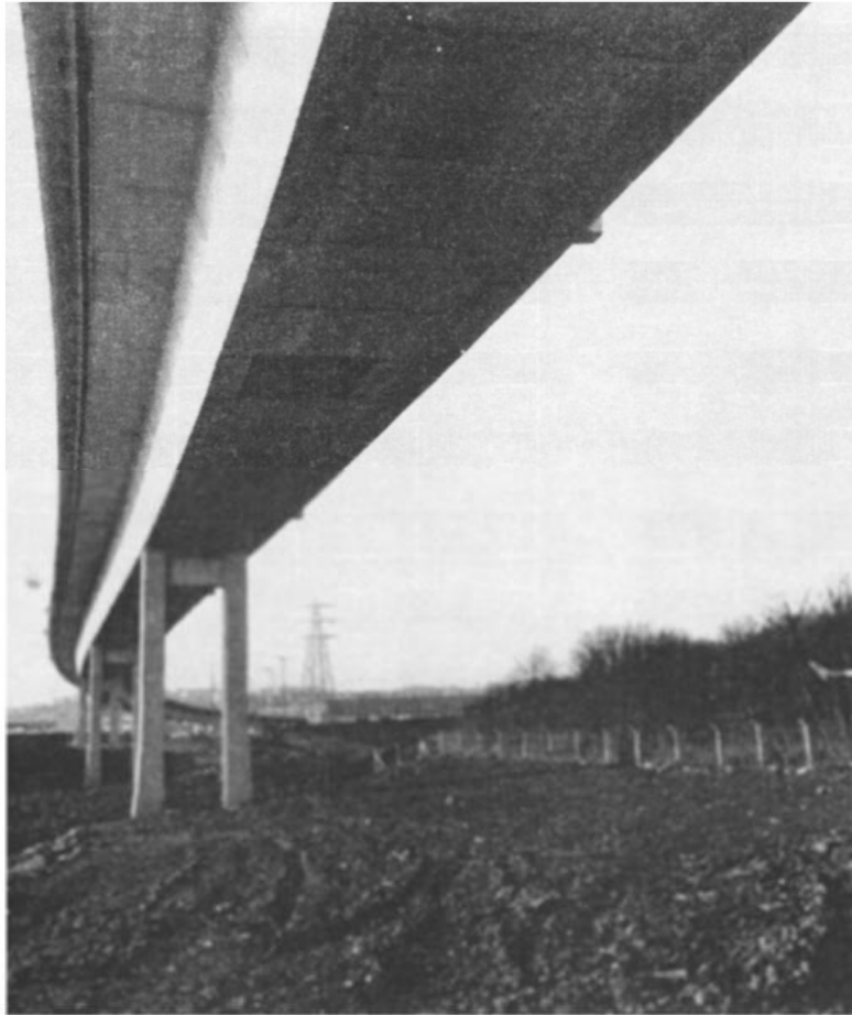
Fig. 1.15 Concrete box girder deck of segmental construction at East Moors Viaduct, Cardiff, Wales; designed by Robert Benaim & Associates. Photographs courtesy of Shepherd, Hill Ltd and Robert Benaim & Associates.
