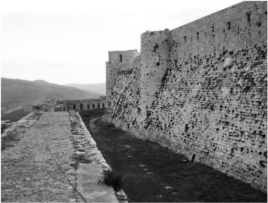
The Crusader castles were built to last – this is the Krak des Chevaliers castle in northern Syria, controlled by the Knights Hospitaller. It fell to Muslim forces in 1271. (Author, Paul Moorcraft)
