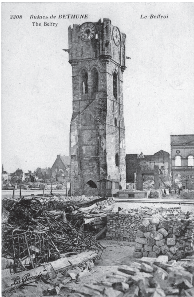
0.1 The damaged belfry at Béthune after the First World War. Before the war there had been buildings surrounding the belfry, and the roof outlines of some of these can be seen. ( Authors' collection )
