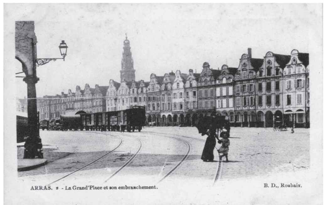
1.7 The standard gauge branch lines in the Grande Place at Arras, with wagons being unloaded onto carts, before the First World War. (B.D., Roubaix; Authors’ collection)
