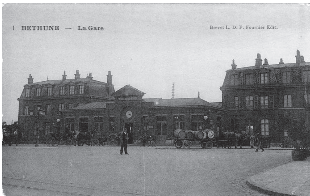
1.9 The Compagnie du Nord station at Béthune, probably before the First World War. The tracks of the metre gauge tramway from Béthune to Estaires can be seen crossing the forecourt in the foreground. ( Brevet L. D. F. Fournier Edit; Authors' collection )
