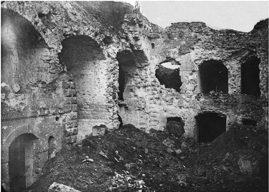
Results of artillery tests at Fort de Malmaison in 1866. (LOC)
