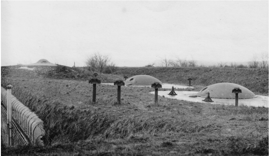
Schumann's design for the 21cm howitzer armoured battery at Feste Manstein, Metz. (NARA)
