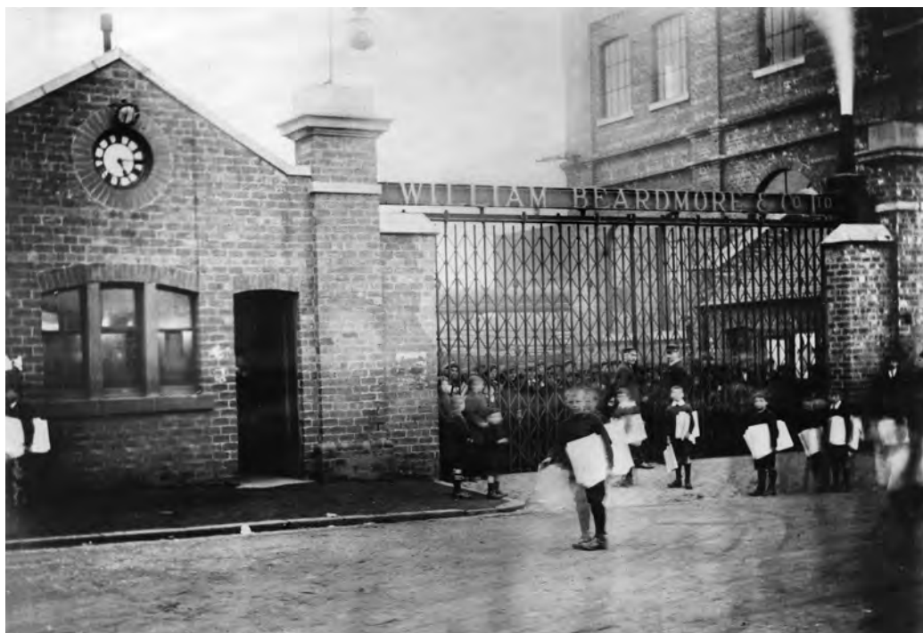
Left: 16 October 1916. The clock is showing 5.14, one minute before the working day is over and the gates will be opened by the gatemen. Tramcars would have been lined up on the main road not far from the yard to deal with this mass exodus. Young boys in the employ of local newsagents wait to sell evening newspapers to the men. During the First World War employment at the Dalmuir works peaked at over 13,000 people. (Author's collection)
