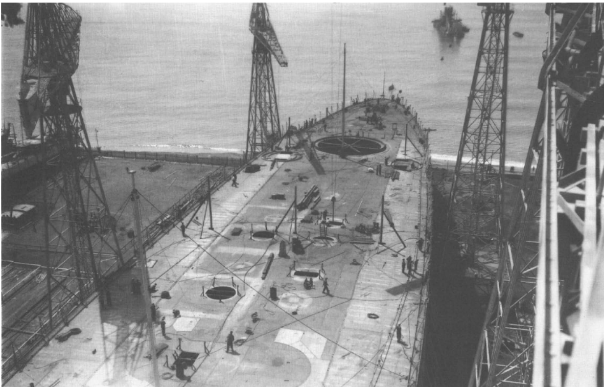
Littorio in August 1937 on one of the ways of the Ansaldo shipyard at Genova Sestri-Ponente; the ship is almost ready to take to the water and the pontoon in the background is working on preparing the foreslip.
