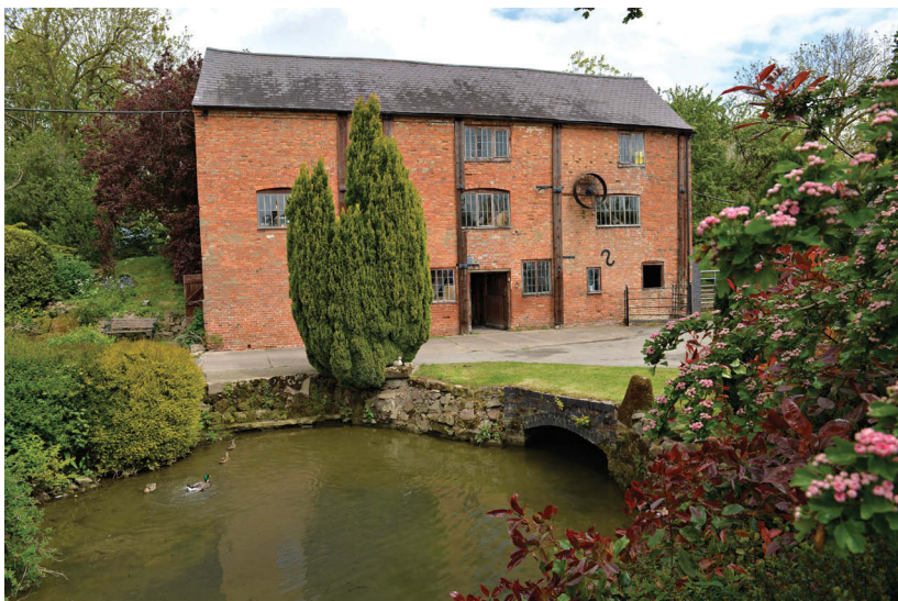
Claybrooke Mill stands on a site where milling has continued for a thousand years. The internal waterwheel is to the right of the building.
