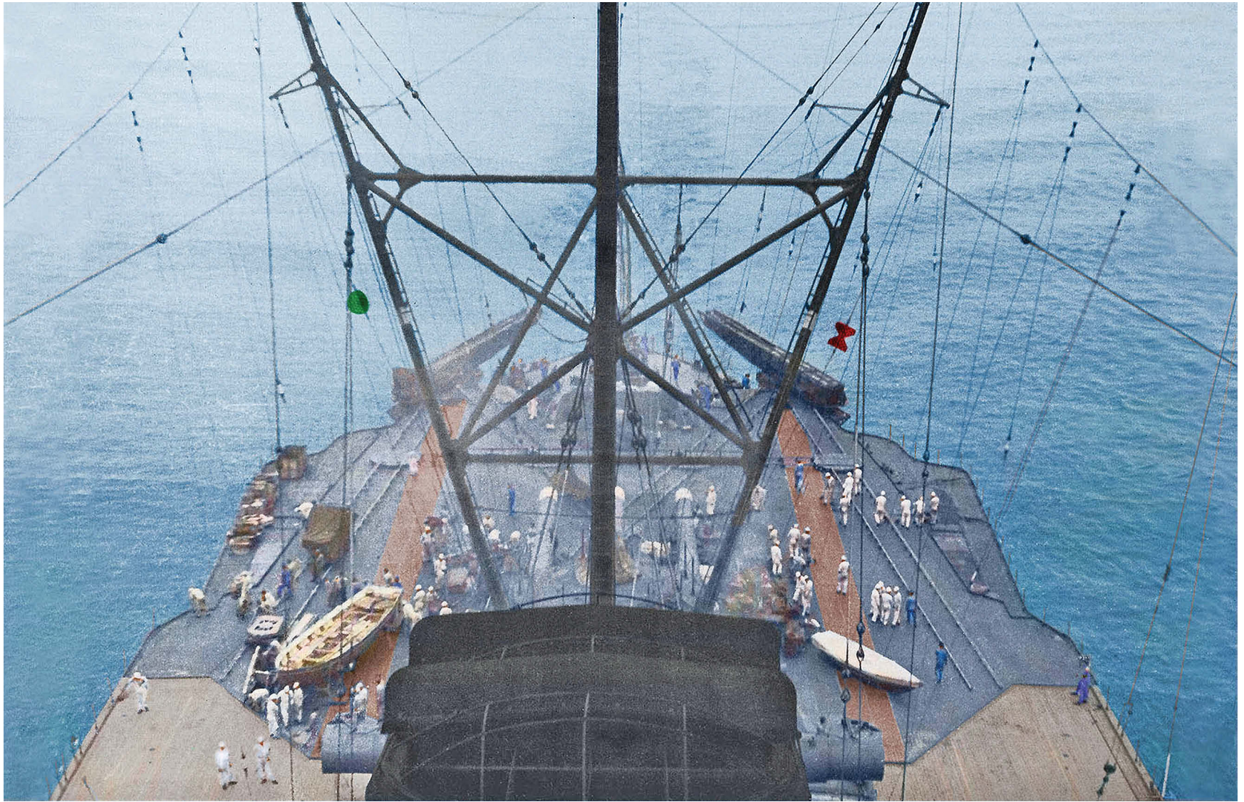
View from Musashi's tower bridge to the funnel, main mast and aircraft deck in May 1942, during finishing works; the two boats visible were fitted only temporarily.
