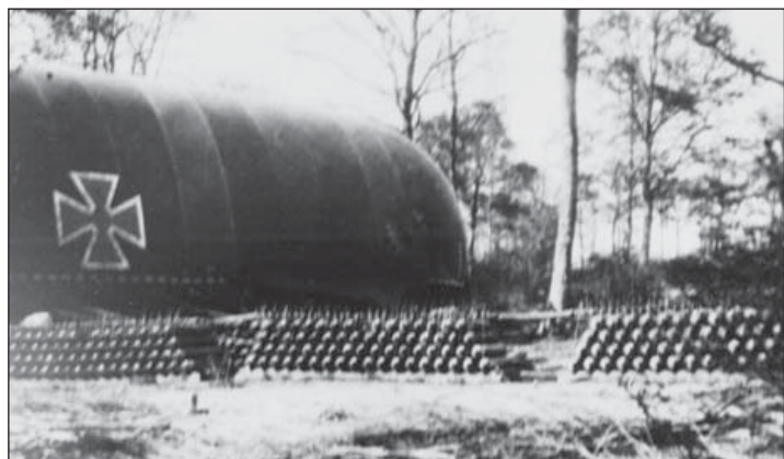
Hydrogen bottles sit stacked and at the ready at a German Ballonzug . Even if they were not set afire, it cost time and money to repair, reinflate and re-raise damaged balloons. If an observer parachuted while under attack and the balloon was unharmed, it would have to be winched down and then sent up again (Tom Darcey Collection via Greg VanWyngarden)
