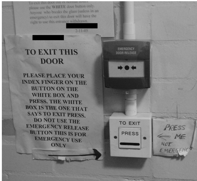
FIGURE 1.3 The presence of three separate formal and informal sets of instructions (and a threat of removal of entitlement of door use!) suggests that something may be amiss with the design of this set of door controls.
