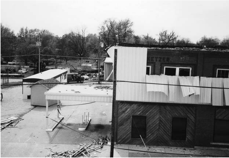
Plate 2.1 Severe wind damage to structure.
