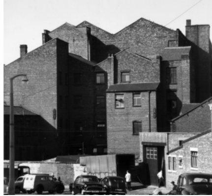
1.1 James Frazer Stirling, photographer, houses in Avenham, Preston, England (1957–61)
