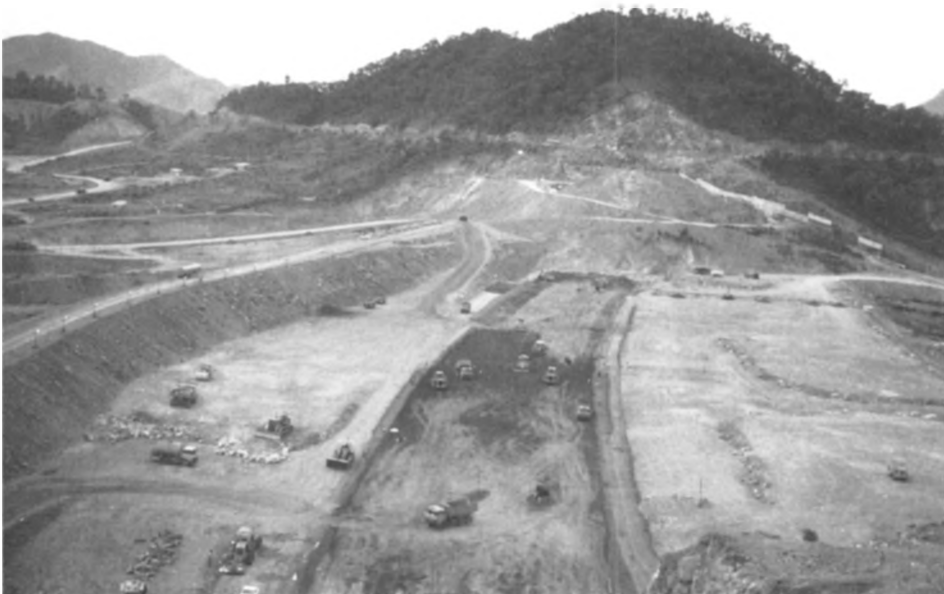
Figure 2.3. Kinda dam, Burma 1983 (courtesy of LI).
