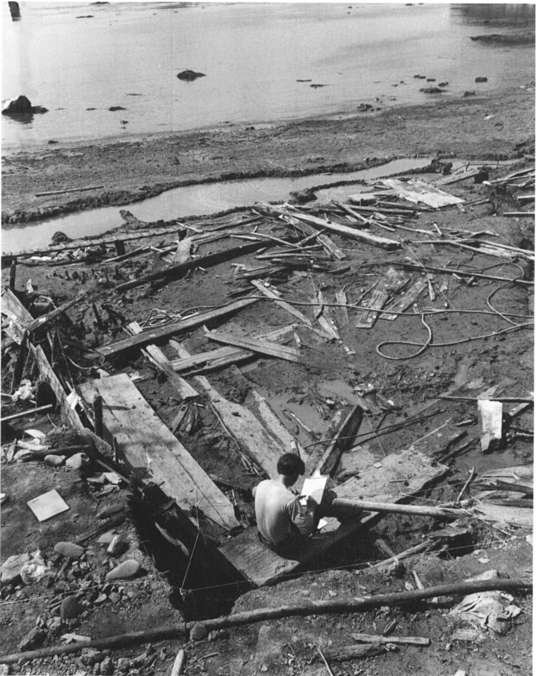
FIGURE 2 Sleeping benches, complete and broken house roof and wall planks, and the lower portion of the south wall of House #1 partially exposed. The pond is a settling basin for sediments washed from the site during excavation, and was constructed by the crew to protect the marine environment of the reef in front of Ozette Village. (Photo by Ruth and Louis Kirk.)
