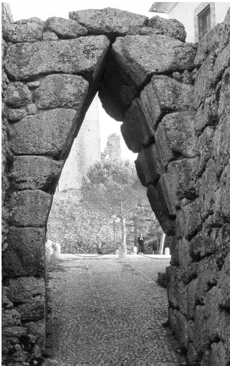
Figure 1.6 Arpinum, polygonal walls and corbelled gate, c. 300 BC.
