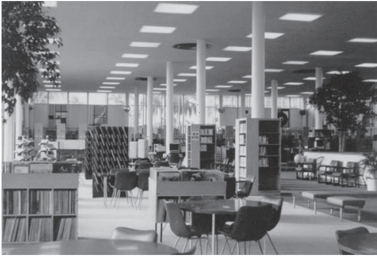
PHOTO 1. West Palm Beach Public Library: Before
