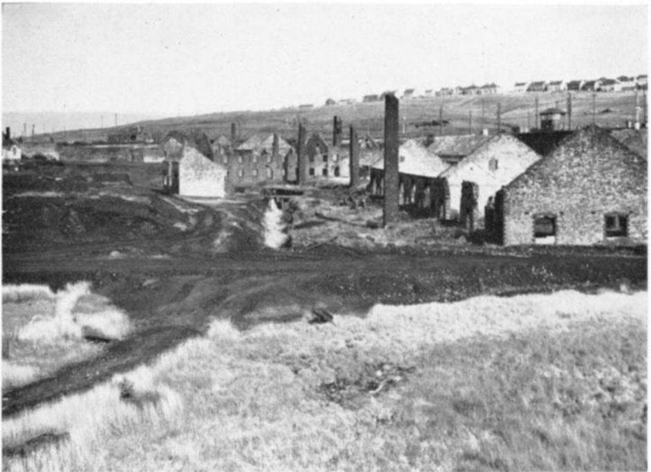
III. Derelict spelter works near Swansea
