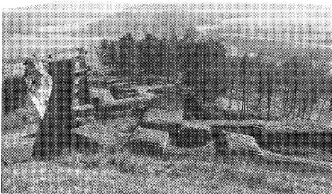
7 Covered way with multiple traverses (Montmédy Citadel). A small re-entrant place of arms is at the left centre
