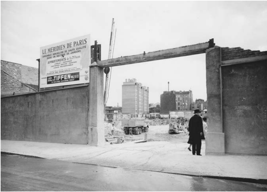
Figure 0.2 Peering into the building site of the future “Méri­dien de Paris” housing development, rue Émile-Dubois, May 1964. Source: Coll. Pavillon de l’Arsenal, cliché DUVF.
