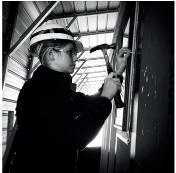
Figure 0.2 Setting the window, 802 LAB, CASA 802, Northfield, Vermont, USA, 2016
