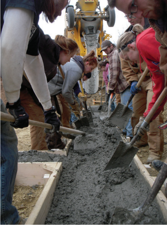
Figure 0.5 Foundations, Studio 804, Lawrence, Kansas, USA
