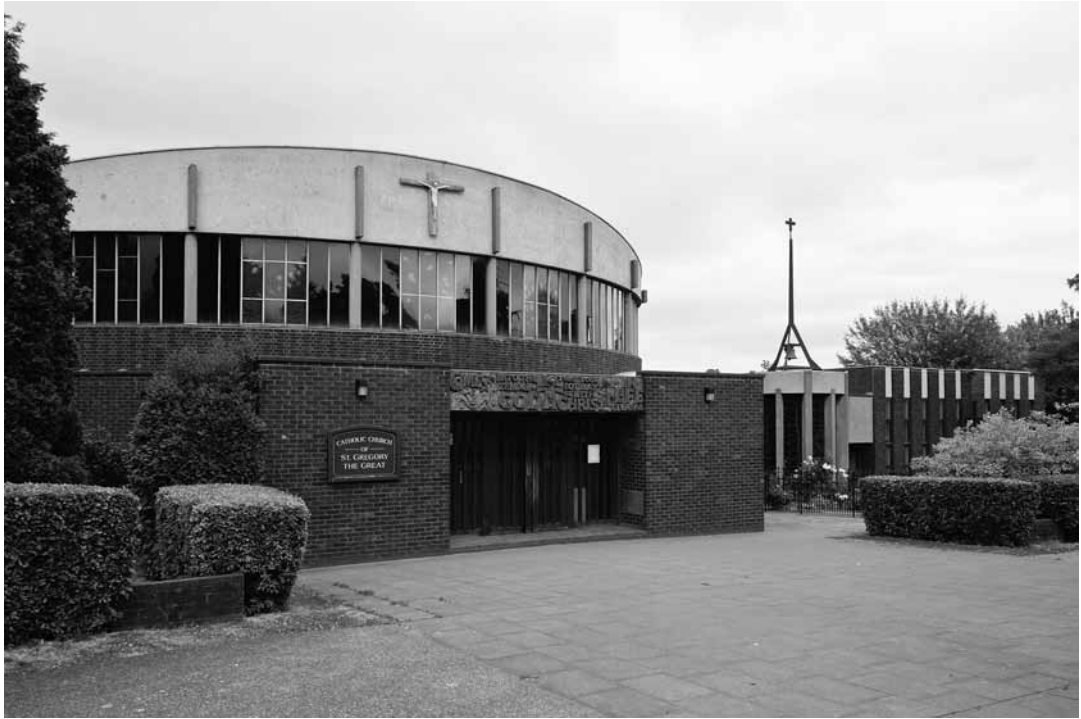
1.2 St Gregory, South Ruislip, London, by Gerard Goalen, 1965–67. View from street: lintel sculpture by Steven Sykes. Photo: Robert Proctor, 2010
