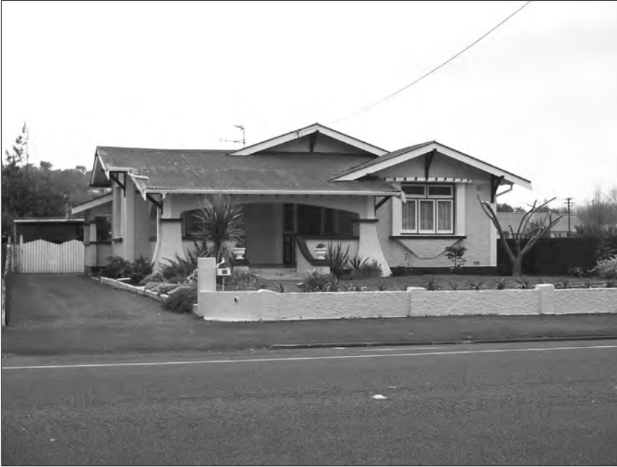
1.2 This 'California bungalow' at 22 Jones Street, Wanganui, was an early 1930s home of Snelling's family, author photograph, ca. 2003.
