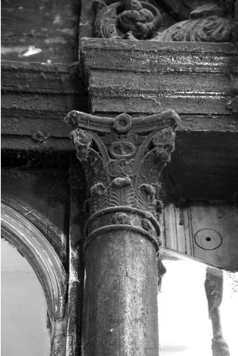
I.7 Ornamental cast-iron capitals in the Galerie Véro-Dodat (1826), Paris. Photograph by Paul Dobraszcyk.
